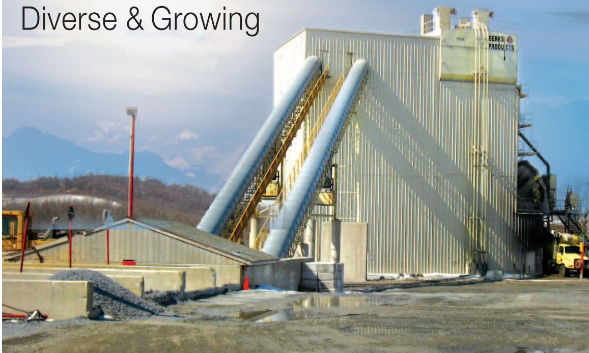
Big Plant On Campus: This CON-E-CO SLP-CM, erected in 1996 by Jay Robinson, is twice the size of most batch plants.
